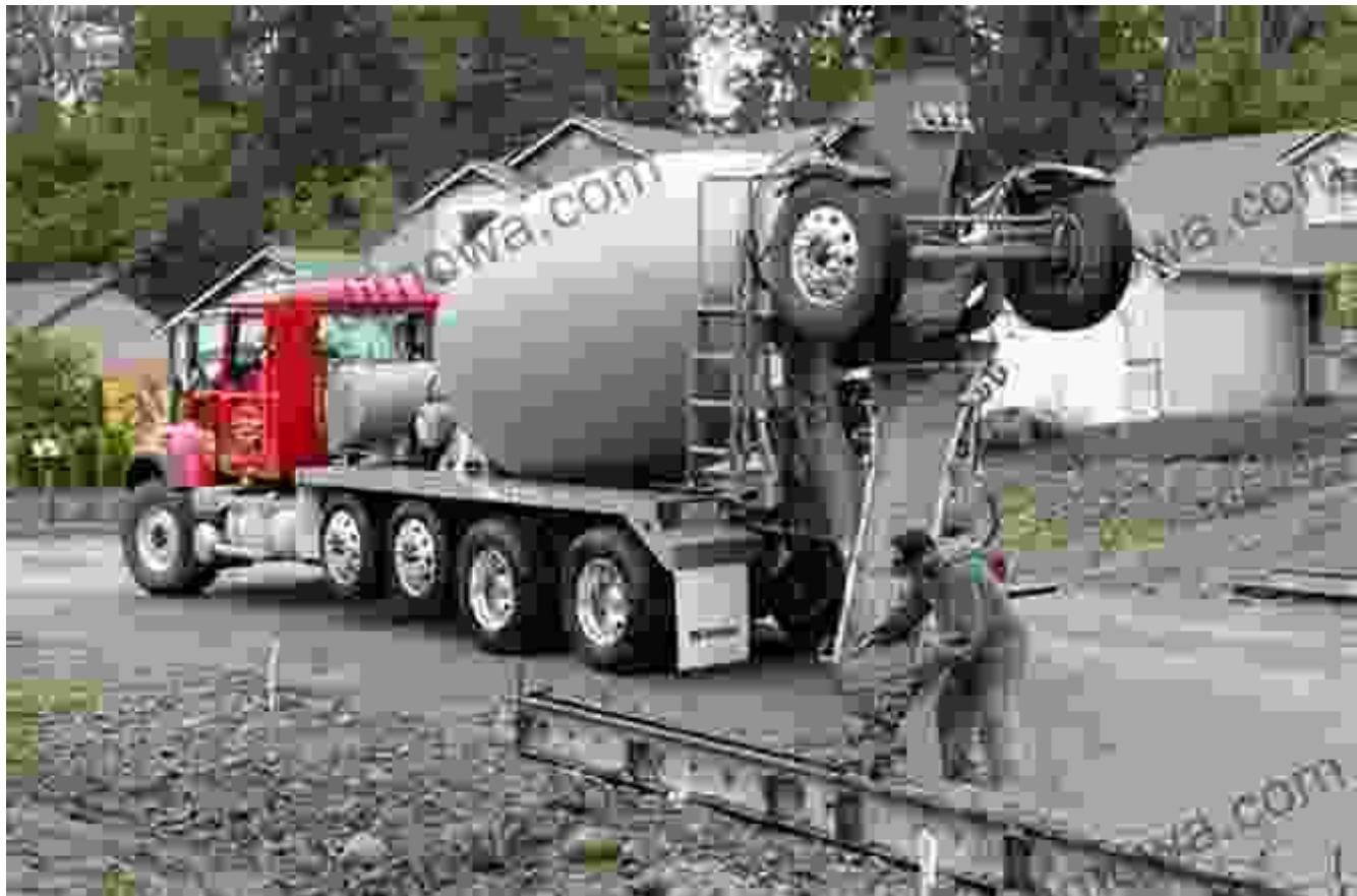
The mixer, a mobile marvel, transforms raw materials into the essential building block of modern structures: concrete. Its rotating drum, equipped with blades or paddles, thoroughly mixes cement, water, aggregates, and sometimes admixtures, creating a uniform and workable mixture that can be poured into molds or directly applied to construction projects.
