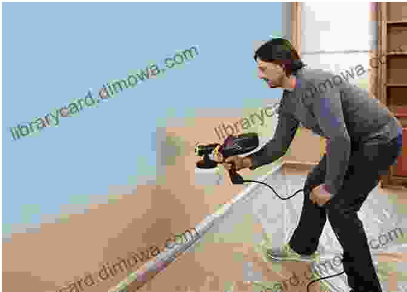
The paint sprayer, an efficient coating solution, seamlessly applies paint, stains, or protective coatings to various surfaces. Its wide range of nozzles and
